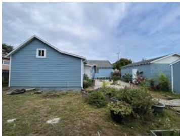
5. WEST ELEVATION - BACK OF PROPERTY
