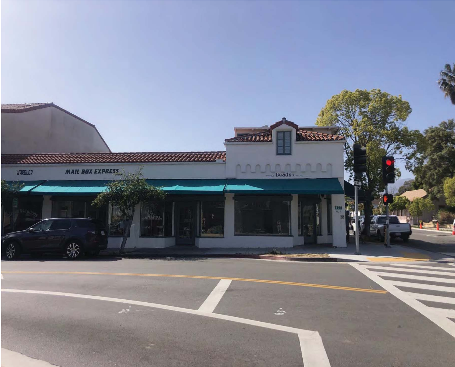
4. View of The Eddy (former Bead Store) from East De La Guerra Steet Facing North (south elevation)
