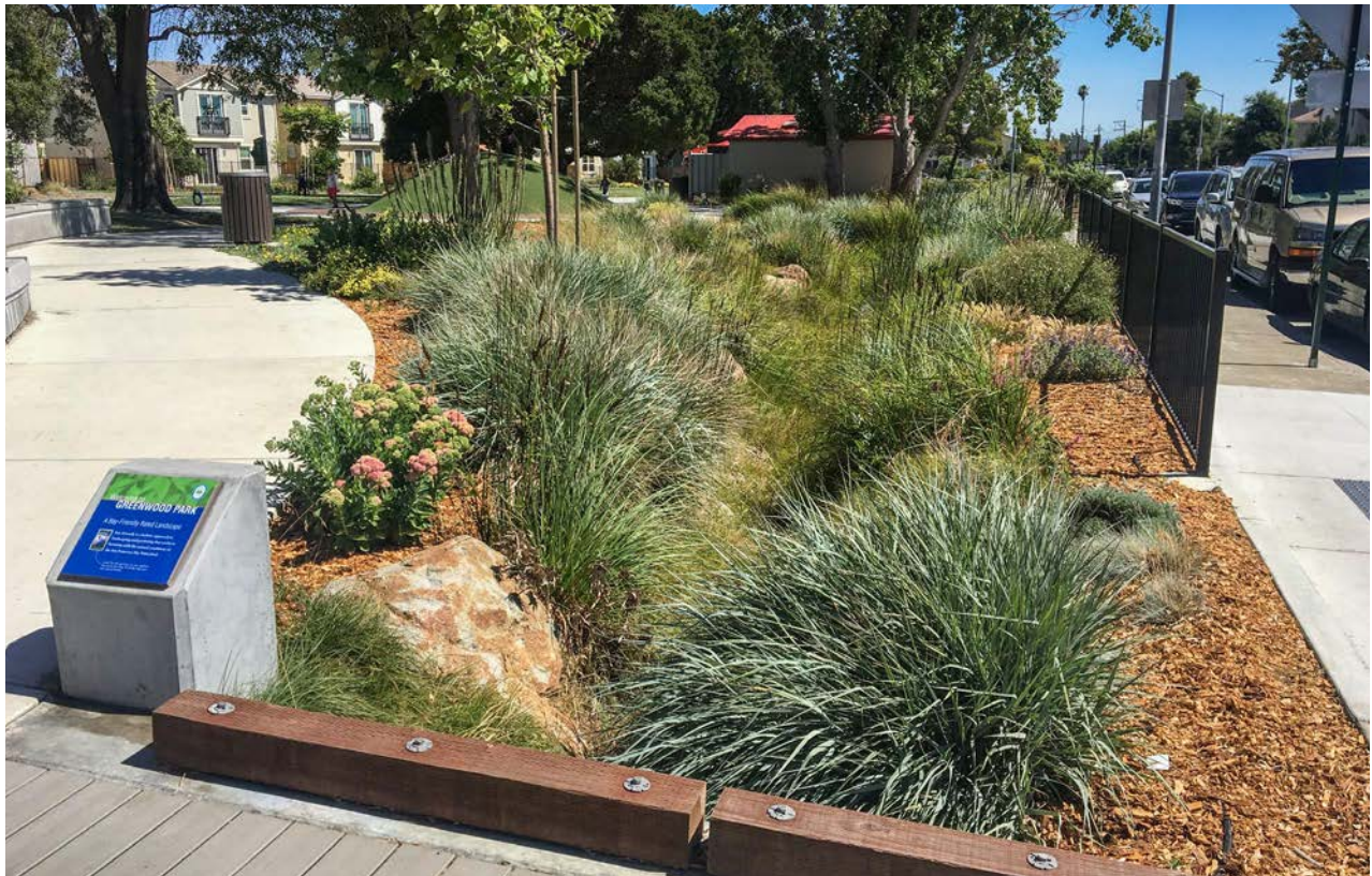
Figure 35: Stormwater Management Area Example
