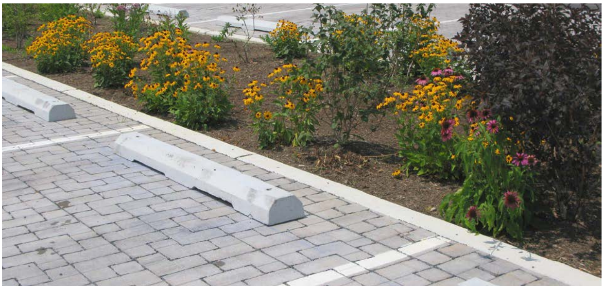
Figure 31: Permeable Vehicular Parking Example
