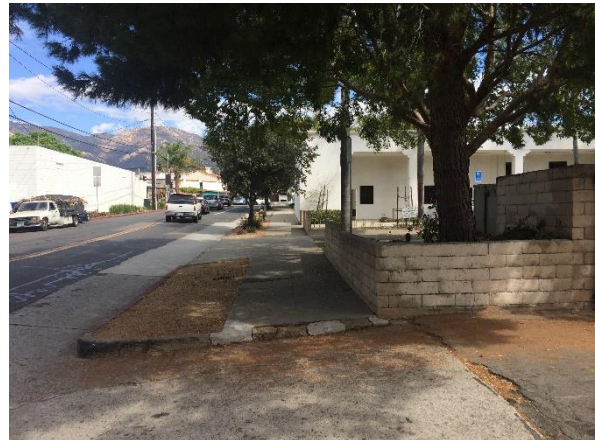
Example of a corner location that needs an access ramp
