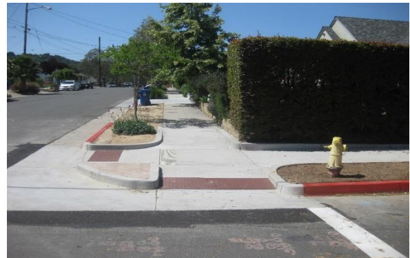
Example of a completed access ramp
