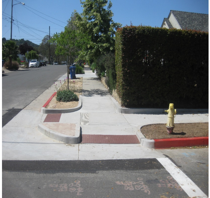
Example of a pedestrian sidewalk access ramp
