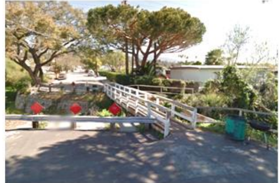
Cacique Street Pedestrian Bridge Before Construction
