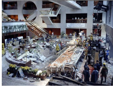
July 1981 Hyatt Regency Collapse
