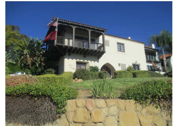
This 1924 Spanish Colonial Revival residence features a wood balcony supported by heavy, carved corbels. The house features the decorative stucco grills along smooth stucco walls that are unique to the Spanish Colonial Revival style.
