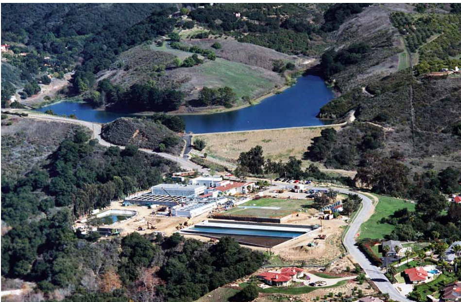
Cater Water Treatment Plant, located in the San Roque foothills
