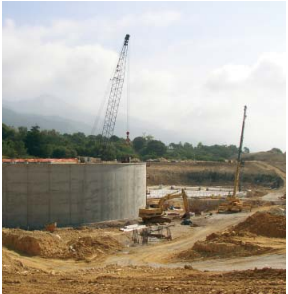
The new Sheffield 6.5 million gallon reservoirs will soon be buried.
