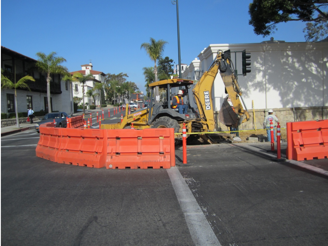
Photo Taken March 4, 2013: Demolition of North East corner of Anacapa/Carrillo Intersection
