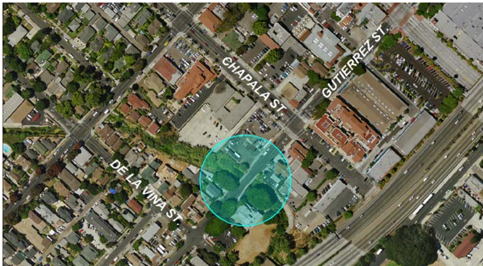
Gutierrez Street Bridge from aerial photo
