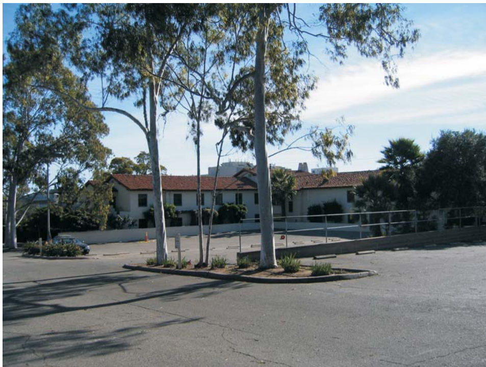
View southwest from public alley toward Knapp Building.
