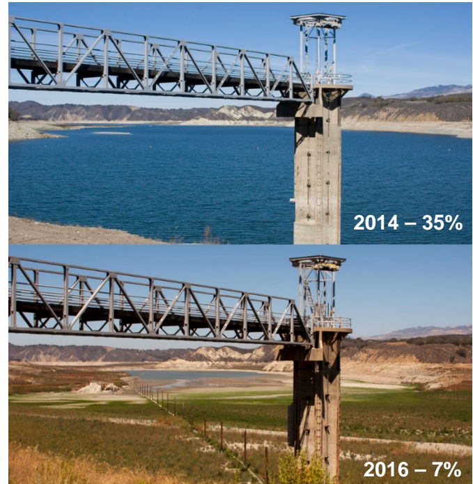
Cachuma Reservoir and intake pipeline for water delivered to the South Coast. Courtesy of the County of Santa Barbara.
