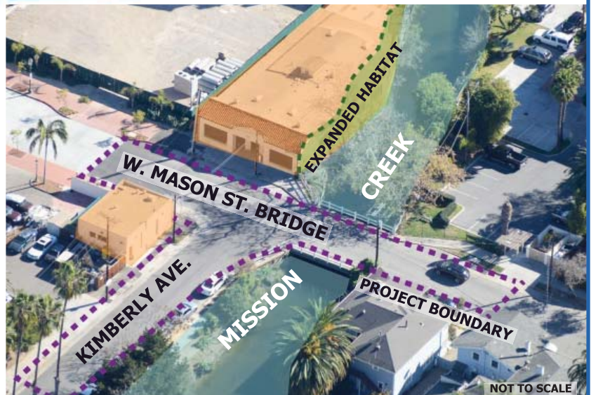
MASON STREET BRIDGE OVER MISSION CREEK BETWEEN STATE ST. & CHAPALA ST.
