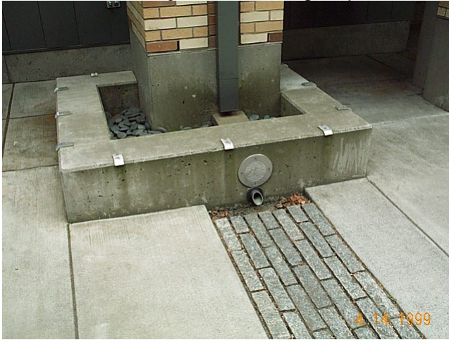
Figure 4-4: Disconnected Downspout Directed to a Pervious Area
