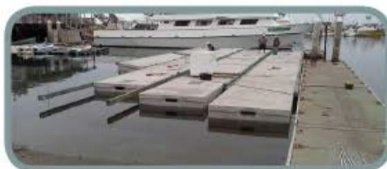
Santa Barbara City Photo: Marina One Construction
