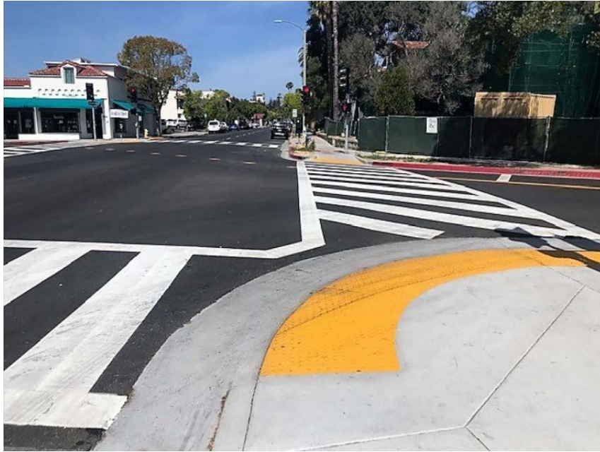
Public Improvements – New Concrete Access Ramps, Curb and Gutter, Crosswalks
