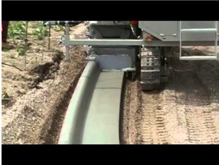
Video by Power Curber 5700-C Pouring Curb & Gutter
