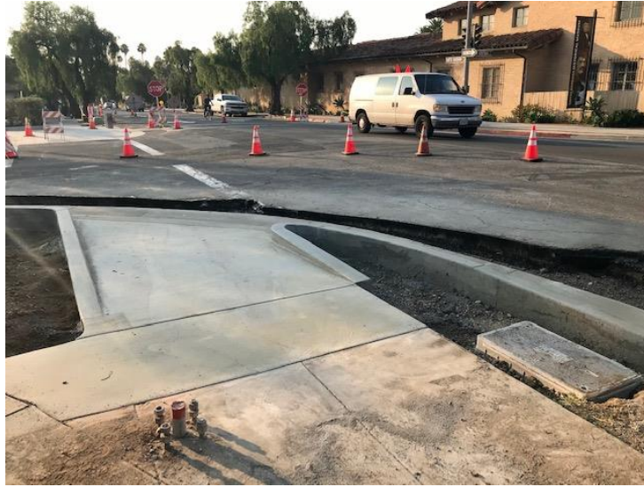
Access Ramp Construction Work on Santa Barbara Street
