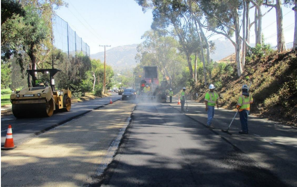
Pavement Grind and Overlay Work on Las Positas Road
