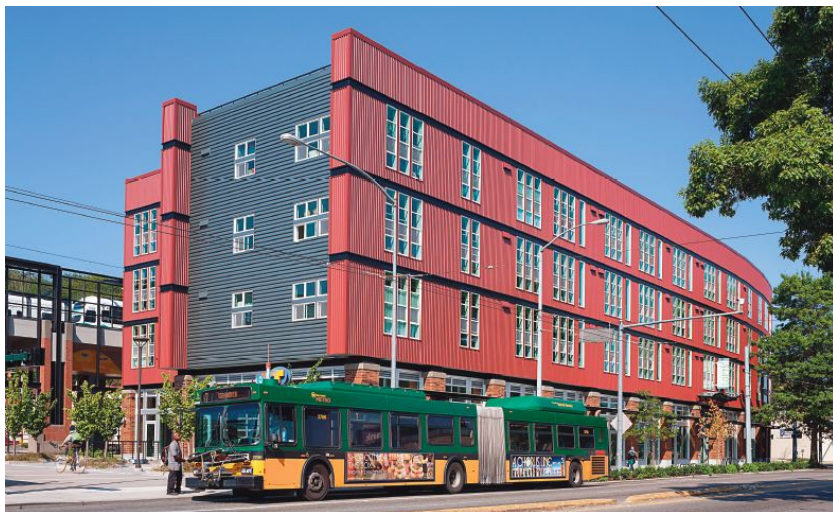
The mixed use transit-oriented development Artspace Mt. Baker Lofts is located on the Central Link light-rail line. It has bicycle storage and a reserved car-share space, but no parking garage. »
