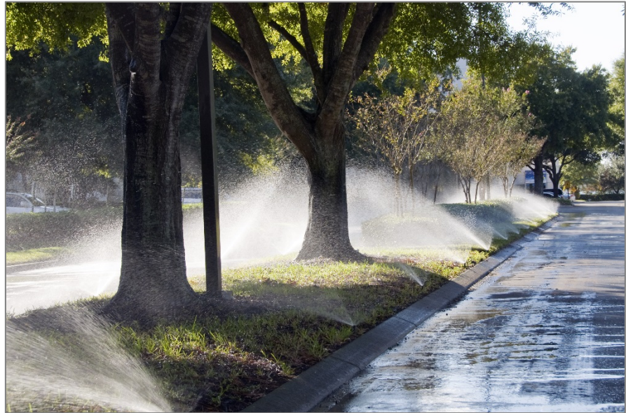
High pressure can cause misting, reducing the amount of water delivered to your plants.
