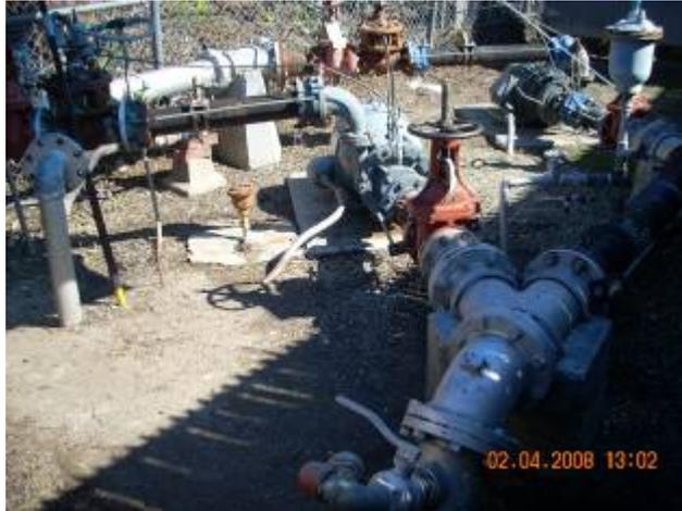
5. Tunnel- located at the Northern end of Tunnel Road. This station will boost pressure to areas of Mission Canyon along both Tunnel and Mission Canyon Roads. There is a 4" green gate valve to pump into and a red Jones hydrant to get water from.
