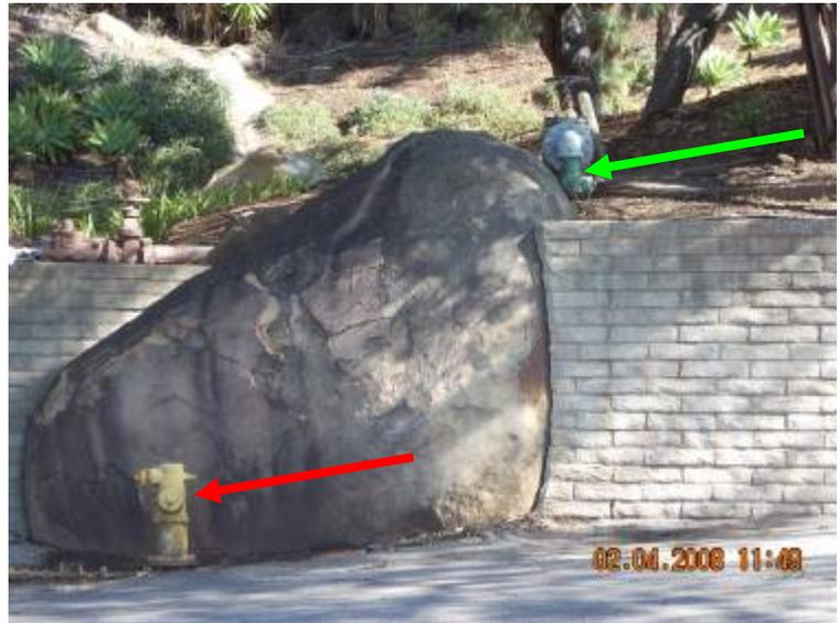
approximately 275 GPM without Fire Department argumentation. The flow may be increased to approximately 475 GPM using the following procedure; Connect to the hydrant at the bottom of the hill at the driveway entrance and pump into the fire department connection located above the large rock near the hydrant. Open the OS&Y valve and pump. Do not exceed 200 PSI and be careful not to collapse the soft suction.
