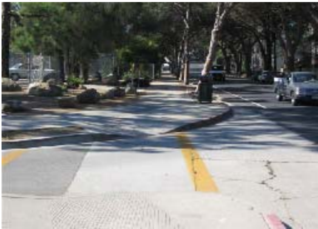
Anapamu at Alta Vista - Before and After
