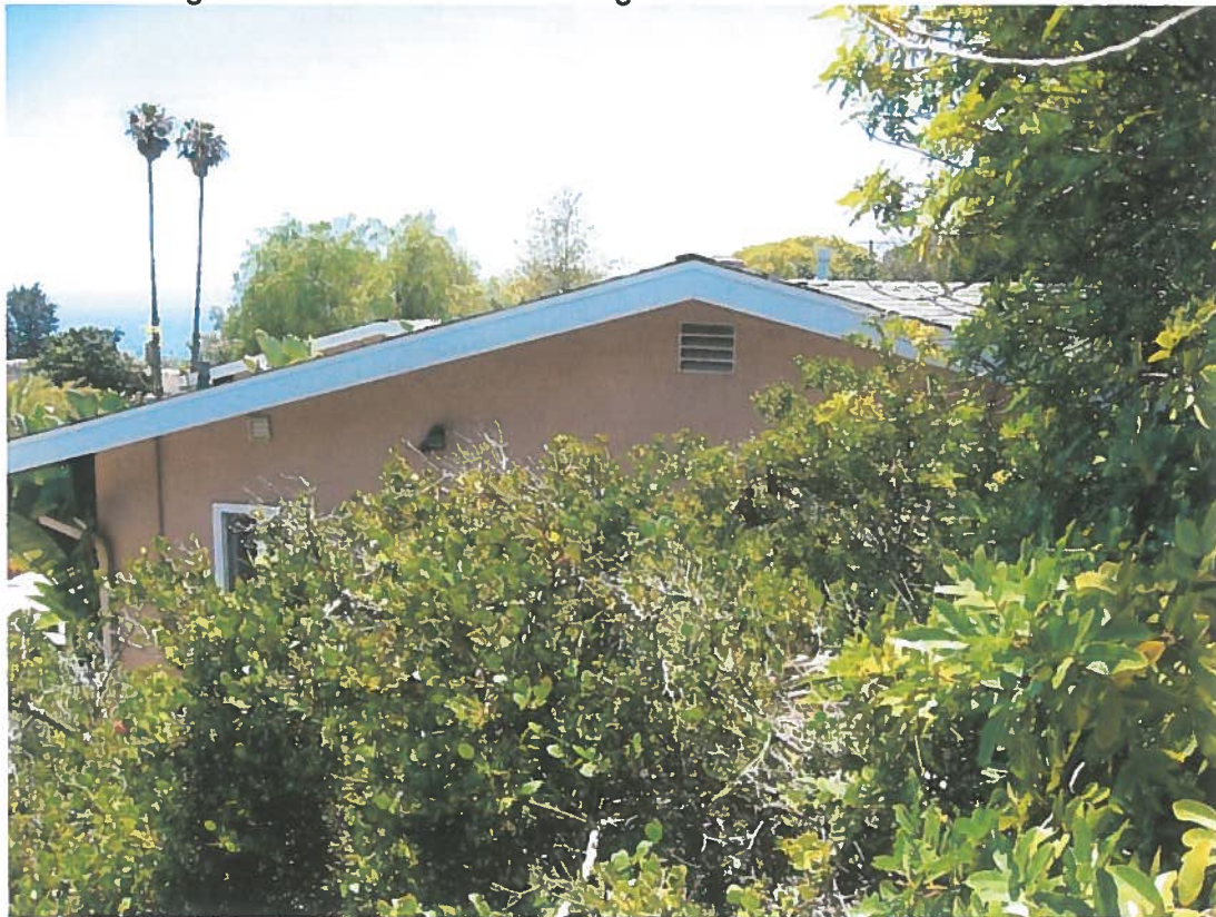
Photo from in front of existing bedroom window (proposed bathroom).
