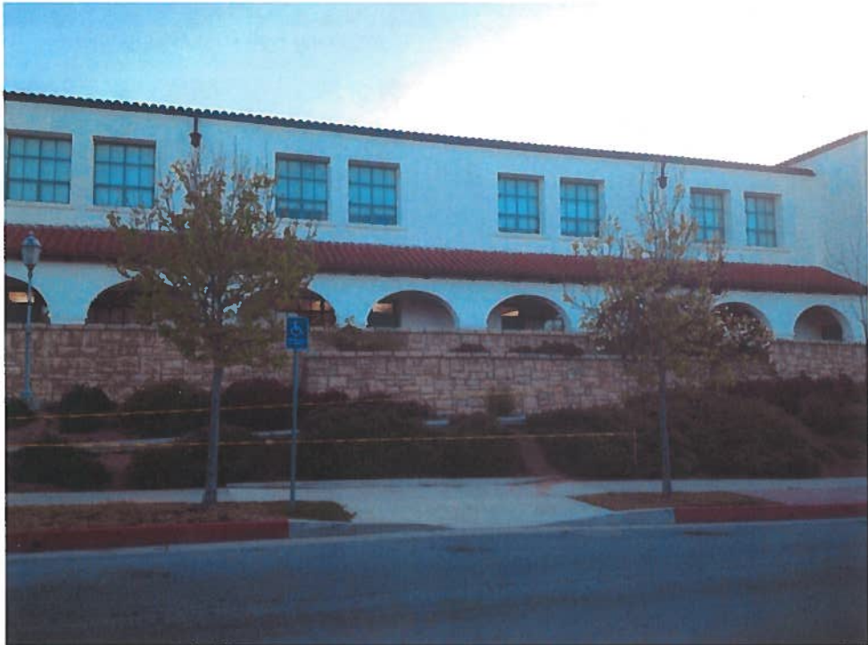
Site walls – New Roosevelt School
