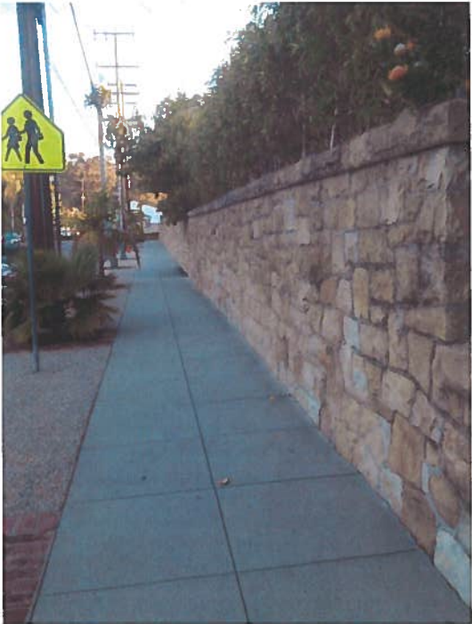
Site wall, back of sidewalk, Mission below Laguna
