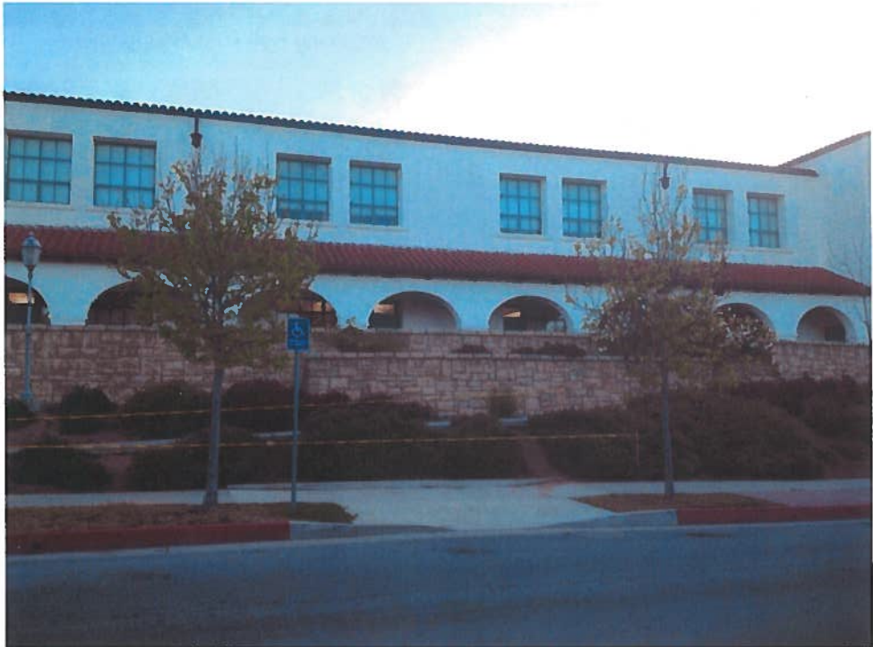
Site walls – New Roosevelt School
