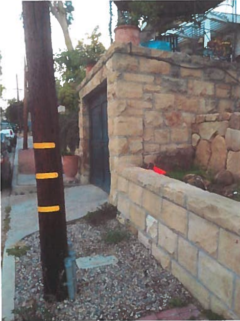
Garage Wall – 1930 Emerson Avenue
