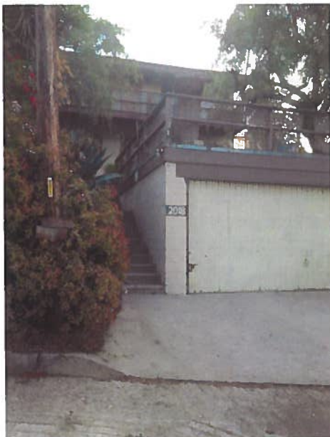
Garage wall – 2018 Emerson
