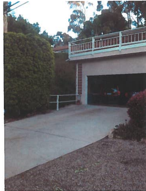
Carport wall & deck - Emerson
