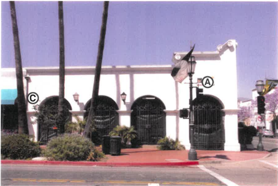
Sign A and C. Photo 2 (looking across State Street)
