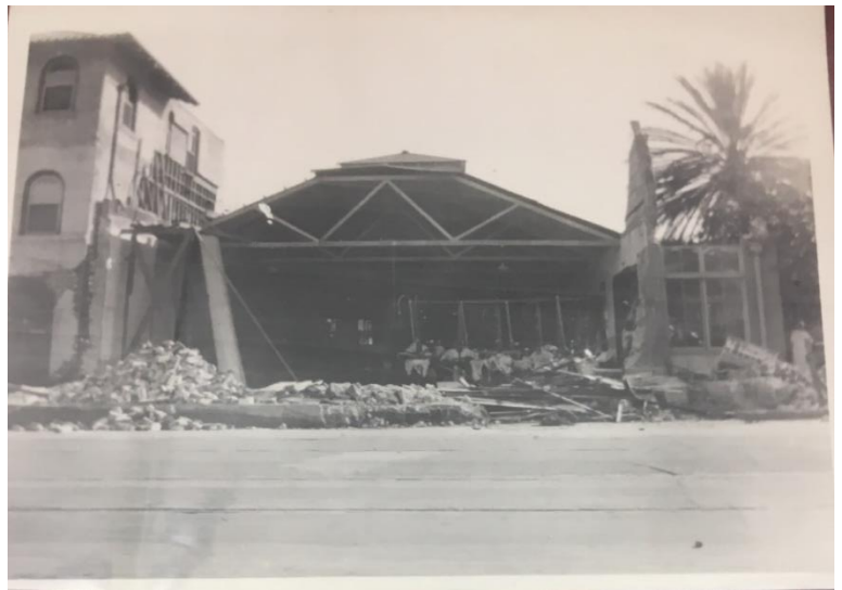
View of building after 1925 Earthquake.
