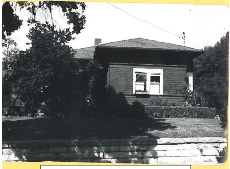
1978 Photograph of the building
