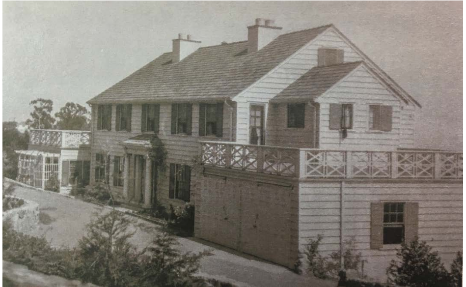
Early photograph of the front elevation.
