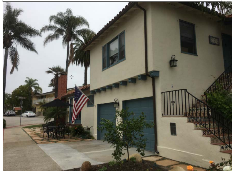
The elevation facing Natoma Street. Photo taken June 2017.
