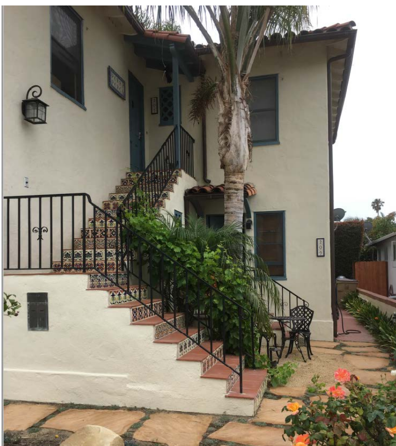
The smooth stucco siding, deeply recessed casement windows, and terra-cotta tile roof contribute to the Spanish Colonial Revival style character.
