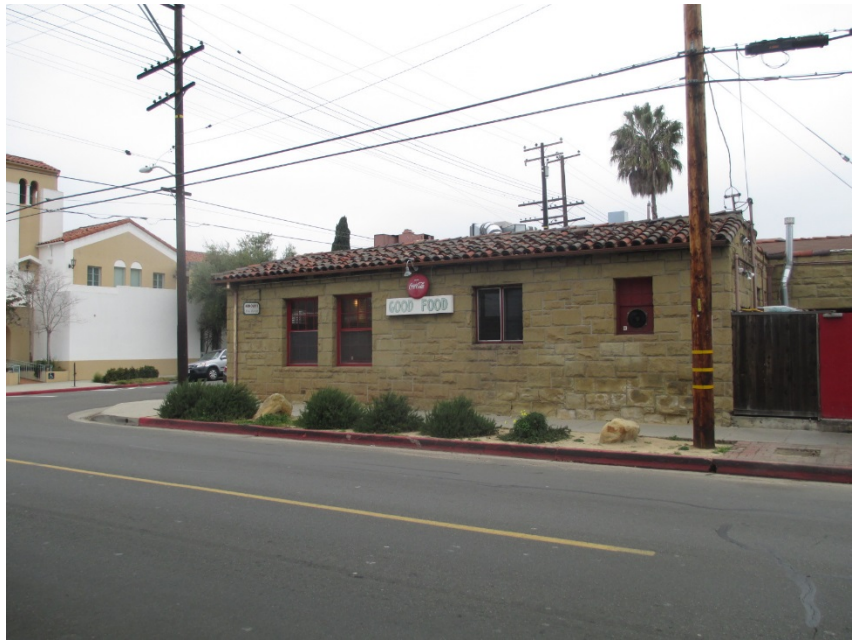
Above: Cota Street elevation of Arnoldi's also has the cut stone walls with deeply set wood windows. Photo taken February 2, 2017.
