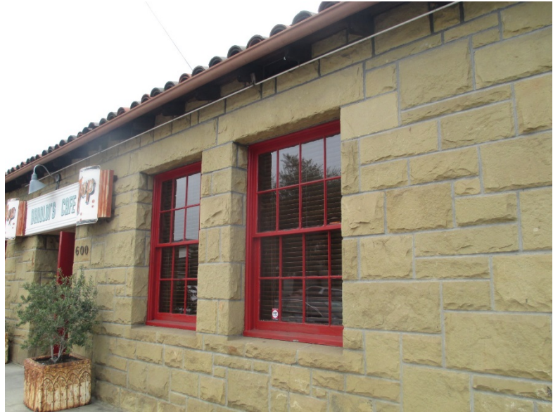
Above: The wood windows are deeply recessed in the thick sandstone wall. February 2, 2016.
