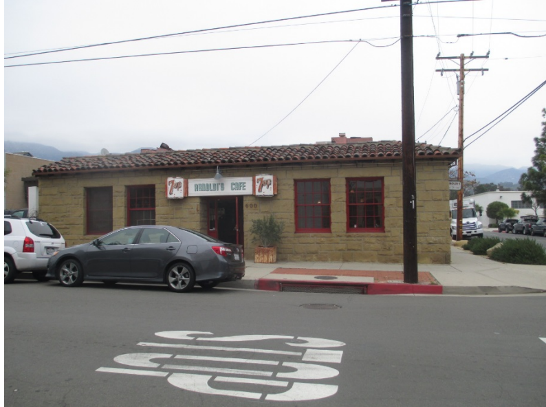
The Arnoldi's restaurant with its distinctive ashlar cut sandstone walls. The stone was quarried and cut by Joe Arnoldi himself. The restaurant has been a center of the Italian culture in Santa Barbara since 1940. Photo taken February 2, 2017
