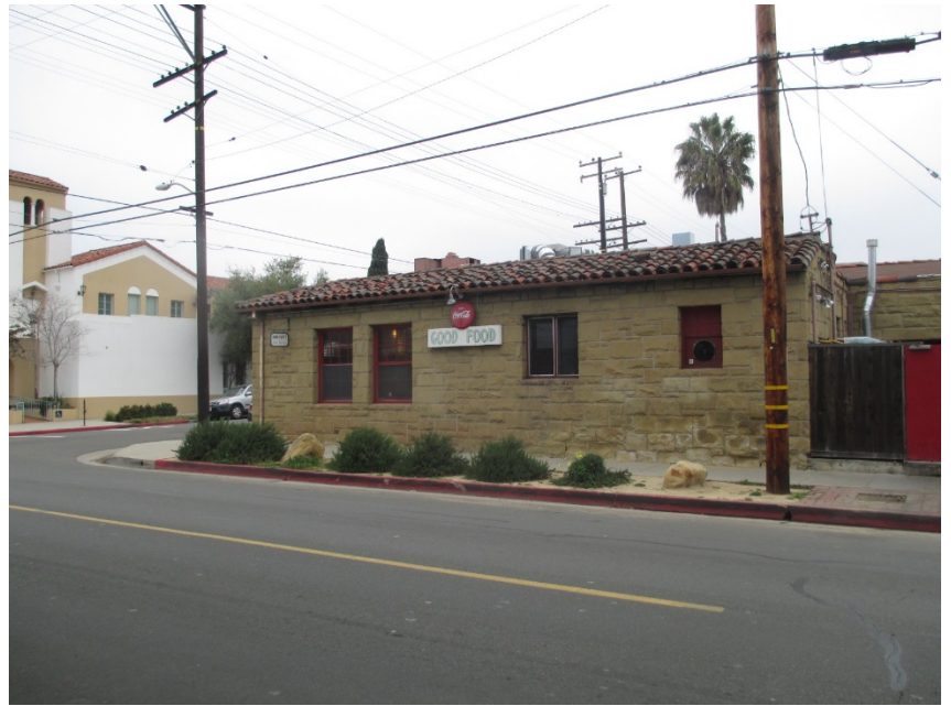
Above: Cota Street elevation of Arnoldi's also has the cut stone walls with deeply set wood windows. Photo taken February 2, 2017.
