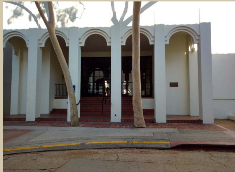
Image: Library South Entrance Prior to ADA Renovation
