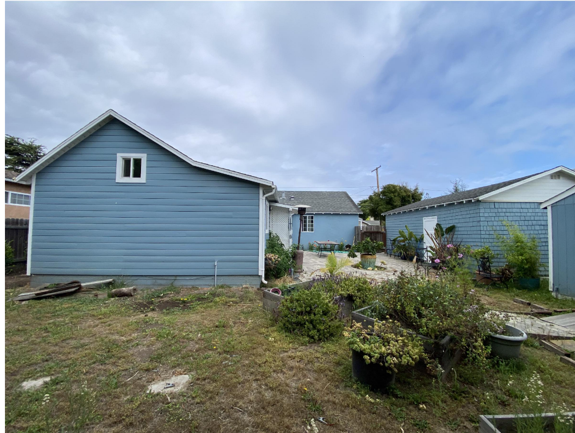
5. WEST ELEVATION - BACK OF PROPERTY
