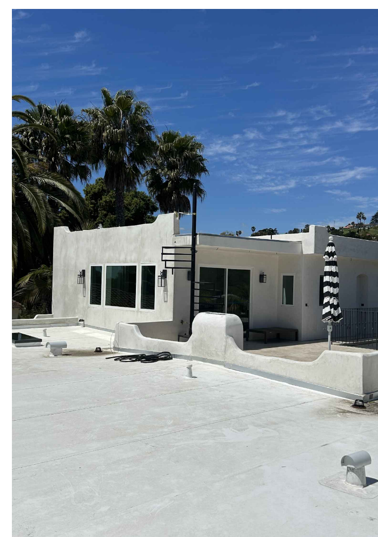
LOWER ROOF LOOKING WEST
