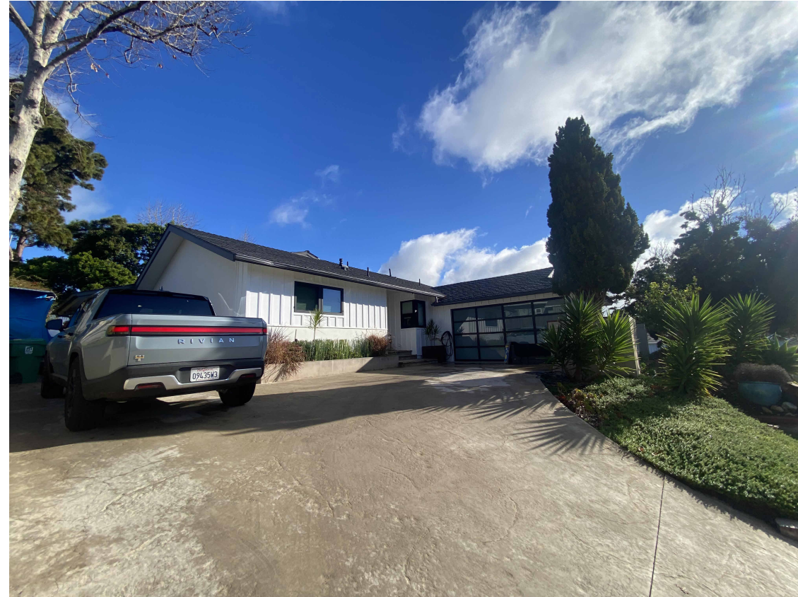
VIEW OF GARAGE AND ENTRY FROM DRIVEWAY
