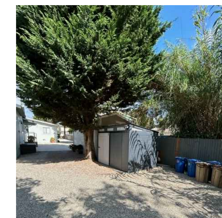
GARAGE AND SHED TO BE REMOVED
