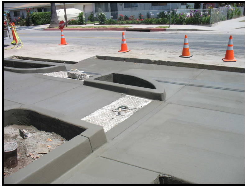
A recently completed ramp, curb and gutter are shown above.
