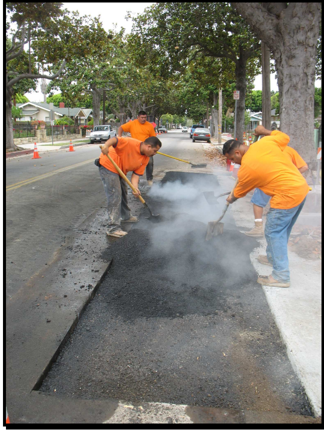
As a last step, the street surface is replaced along the gutter and the curbs are painted.
