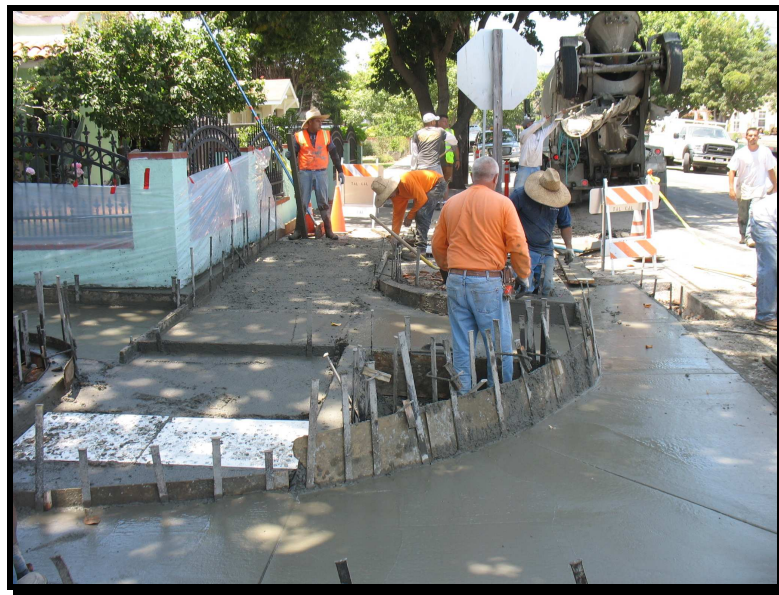
The photo above shows the forms that hold the concrete in place to construct the access ramp and adjacent sidewalk. Notice in this picture the curbs and gutters have been installed.
