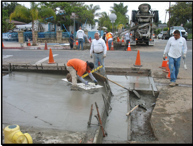
The crew pours the concrete, positions the "detectable warning surface" pad and finishes the access ramp so it ties seamlessly into the street surface.
