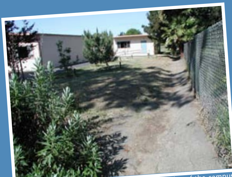
BEFORE: An asphalt drainage ditch along the edge of the campus.
