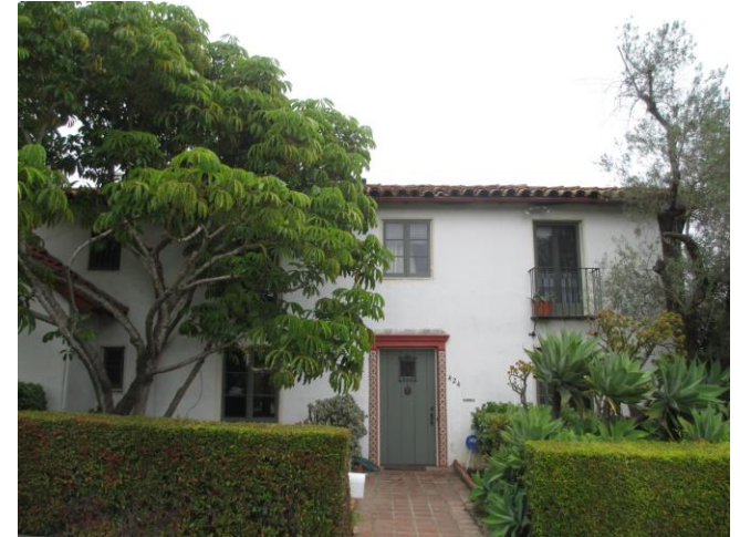
The 1925 house is one of a group of Spanish Colonial Revival residences designed by Mary Craig on the 400 block of Plaza Rubio.
