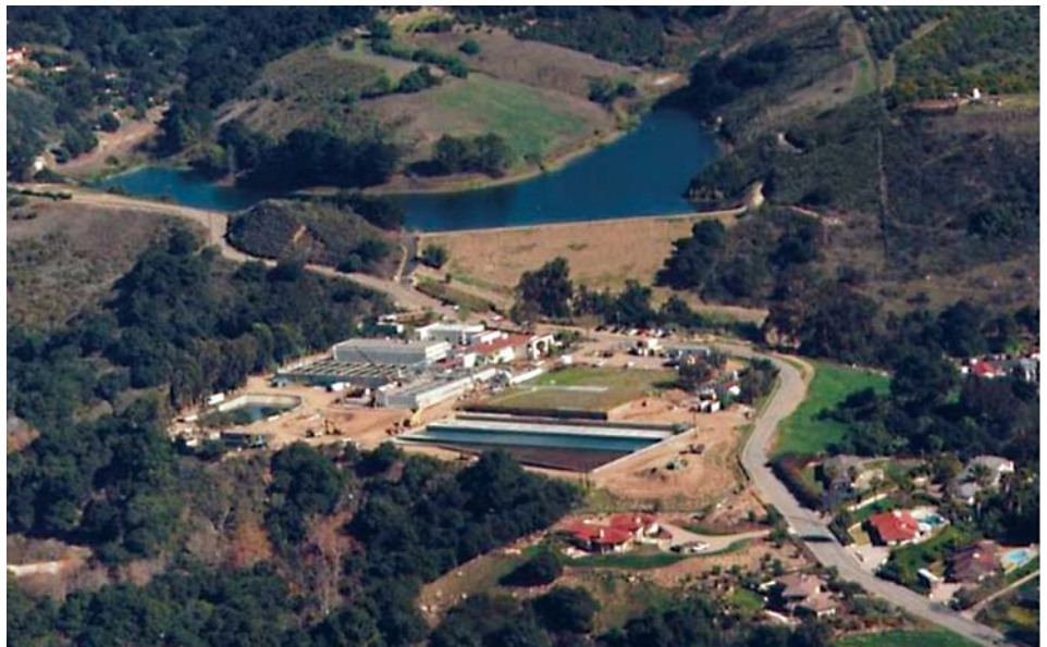
Cater Water Treatment Plant Improvement and Upgrade Project is complete.
