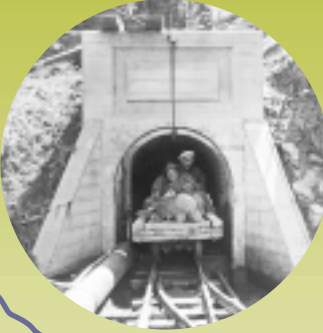
Building the Mission Tunnel The photo below shows the north entrance to Mission Tunnel. It took 9 years to build and was completed on December 21, 1912.
