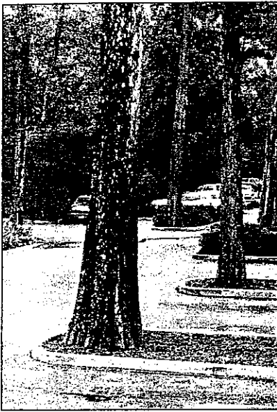
PHOTO 8.5 Excavation into the roots of this tree was avoided by placing the pavement section on top of existing grade and constructing the curb on top of the pavement (see Figure 8.5 for construction detail). (Photo courtesy of Howell Beach, Robert E. Marvin & Associates.)
