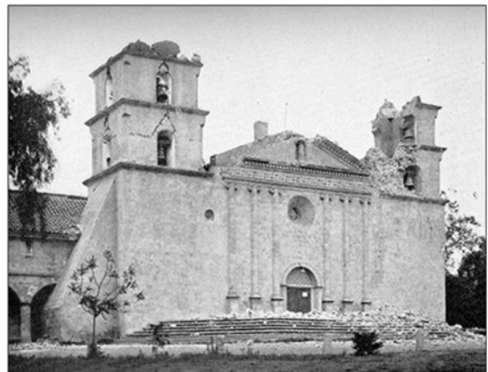
The Santa Barbara Mission was damaged by the 1812 earthquake and rebuilt by 1820. The 1925 earthquake caused the extensive damage shown in this photograph.
