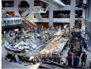
July 1981 Hyatt Regency Collapse
