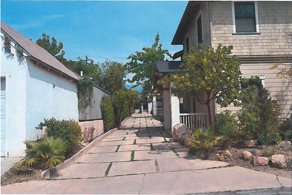
Additions is approximately 1' – 9" from property line "As-built" Laundry Addition at rear of house
