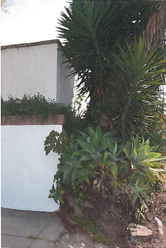
Close up of 10' – 6" corner of wall
