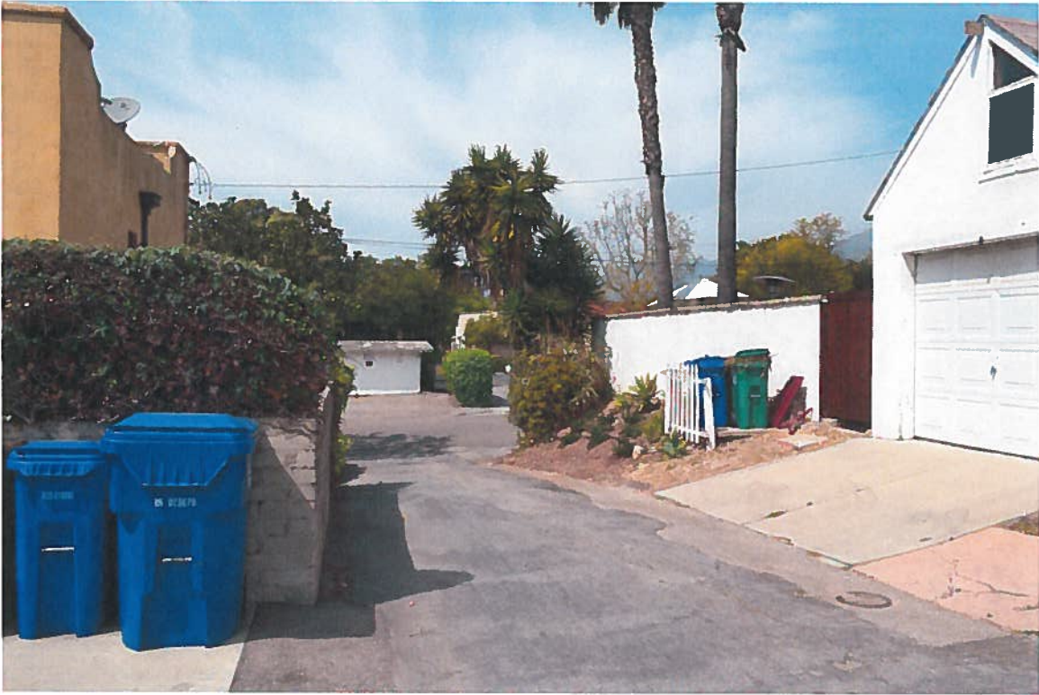
Alley view of as-built site wall
