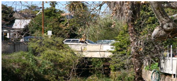
View of Ortega Bridge from Downstream
