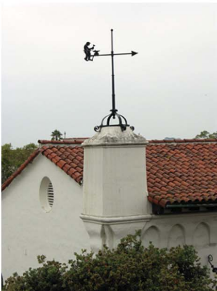
SB Roof Architecture.jpg
