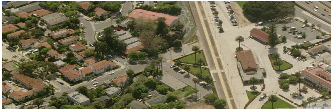
Chapala Street Bridge from Aerial Photo (bridge is left center)
